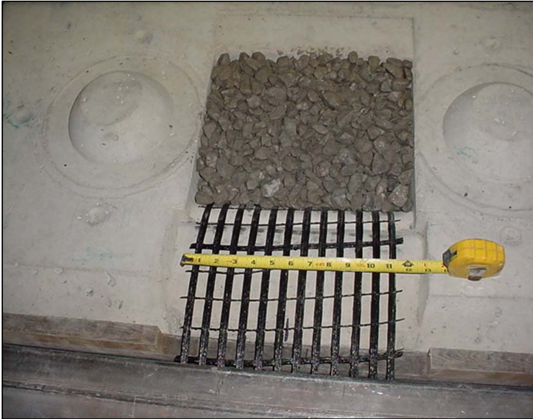
Figure 3: Photograph of the Redi-Rock Positive Connection (PC) Block system and Miragrid 20XT geogrid
