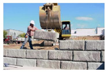
Place an 18 inch x 12 inch (457 millimeter x 305 millimeter) piece of non-woven geotextile fabric in the vertical joint between the blocks to prevent the drainage aggregate and backfill material from migrating through the vertical joints between blocks. (Figure 11)
